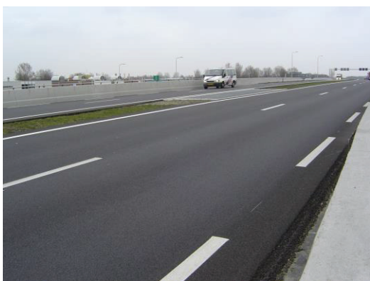
Example application of two layer porous asphalt (Twinlay M) on a provincial road: The N302 at Harderwijk (including the BrainJoint as a jointless joint)
