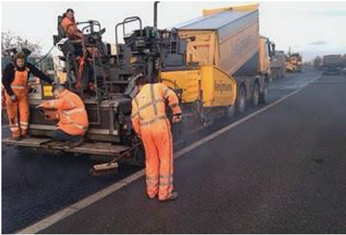
Paving Self healing ZOAB + on the A58 near Vlissingen and the first healing action after three years
