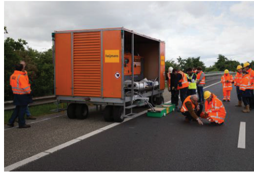
Paving Self healing ZOAB + on the A58 near Vlissingen and the first healing action after three years
