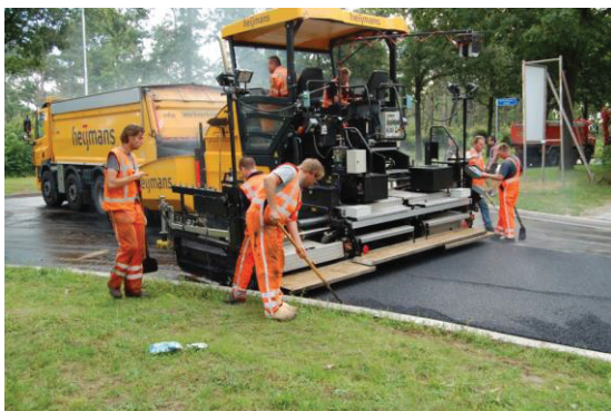
Self Healing Microflex being applied on the intersection crossing area of the Grootvenstraat in Tilburg
