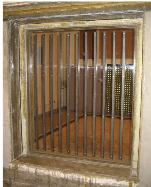
Figure 1. PMMA plate with 11 steel L30 stiffeners attached.
