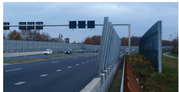
Fig. 6: Noise barriers and "super quiet" asphalt In Harderwijk (photo: P. Driessen)
