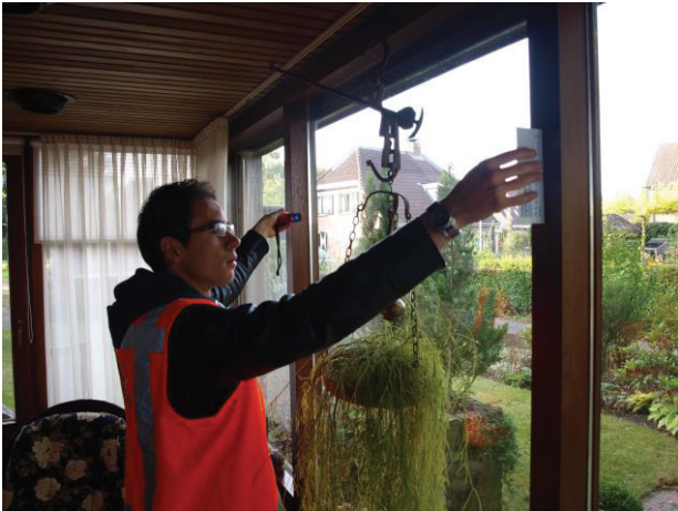
Fig. 10: Taking measurements for replacement window, applying extra noise reducing glass (photo: P. Driessen)
