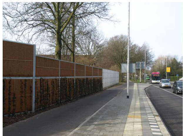
Fig. 9: Example of noise barriers in a residential area (photo: P. Driessen, location Bommel)
