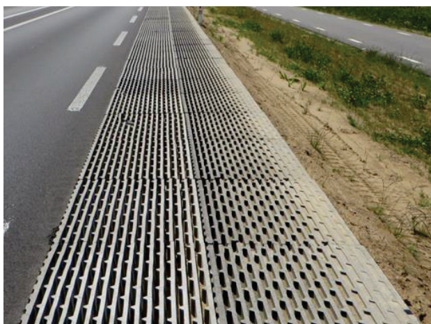
Figure 2. Whisstone diffracting elements variant 2 (section 2)
