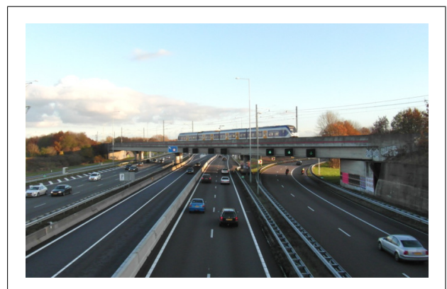
Figure 1. Current railway bridge over the A1 at Muiderberg.
