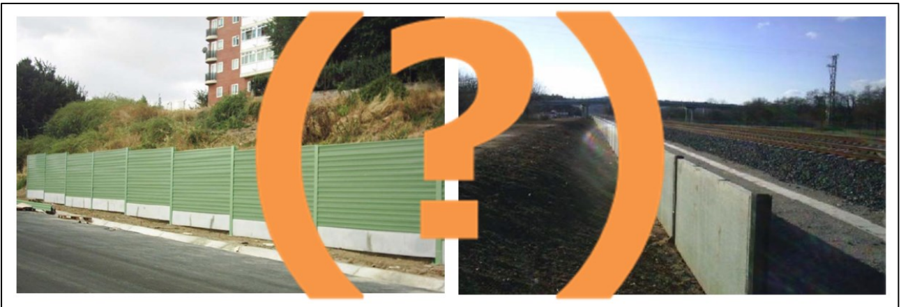
Figure 3. Errors in the location of the sound barrier.
