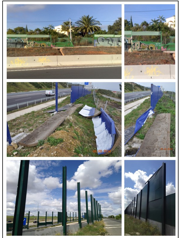
Figure 5. Effects of wind loads on noise barriers in Portugal and in Spain's A8 and M50 highways, assessed by calculations.
