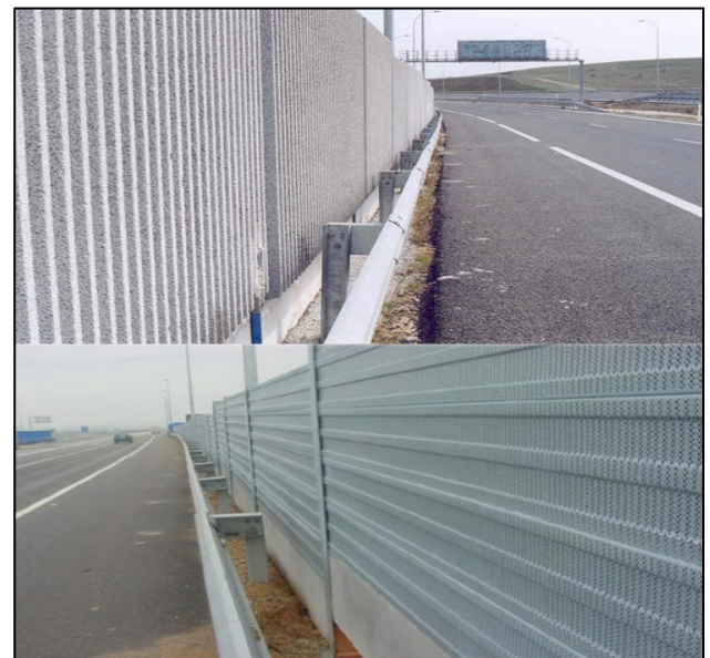
Figure 4. The acoustic barrier prevents proper operation of the safety barrier.
