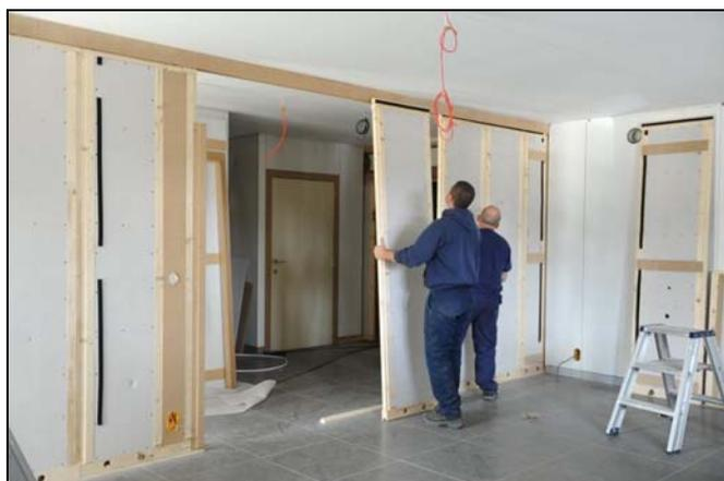
Figure 12. Mounting of interior wall (picture by courtesy of Atelier de l'Avenir)
