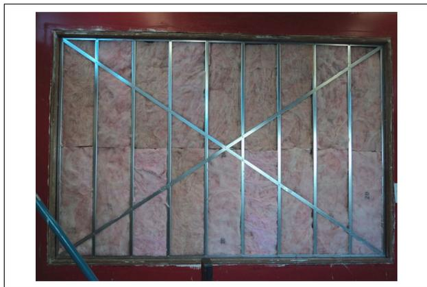
Figure 1. Reference wall assembly in test frame, with sheathing removed. The flat strap cross and bridging channel in the center of the wall brace against lateral and shear loads.
