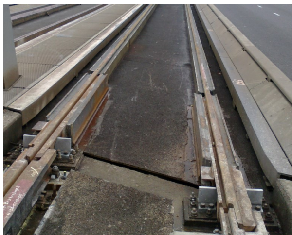
Figure XI: Noise control measures during track renovation. Top left: Diagonal rail joint based in concrete; top right: added mass and stiffness at joint 4; Below : added stiffeners at joint 4, left without rails, right with rails and cork rubber embedding and seatings for bascule bridge rails.
