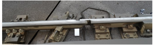
Figure V: Rail joint 4 with from left to right: suspension support, seating support, 2 clamp supports with railpads and far right, embedded rail. The rail on the left moves with the bascule bridge and 'lands' on the seating support which is on a concrete base..
