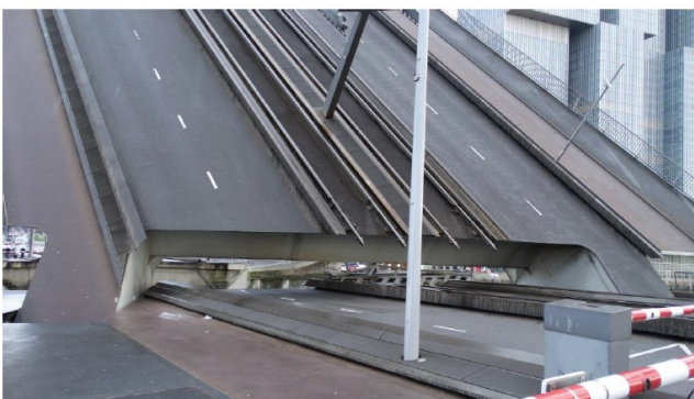
Figure IV: Open bascule bridge with protruding rails. 'De Rotterdam' building is visible on the right.
