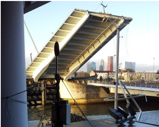
Figure III: Open bascule bridge, northward view, showing main bearing girders and bridge deck with stiffening profiles.
