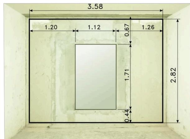
Figure 2. Position of the opening in the dividing wall.
