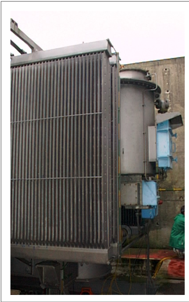
Figure 1. Close picture of transformer tank, showing nearby wall, transformer equipments and radiators.
