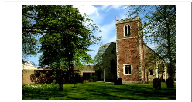
Figure 5. External view of St Margaret's Church (NCEM) [10]
