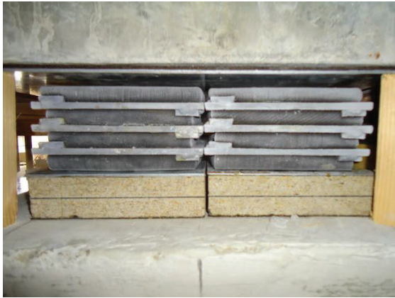
Figure 8. Picture of the installed frozen VHS bearings
