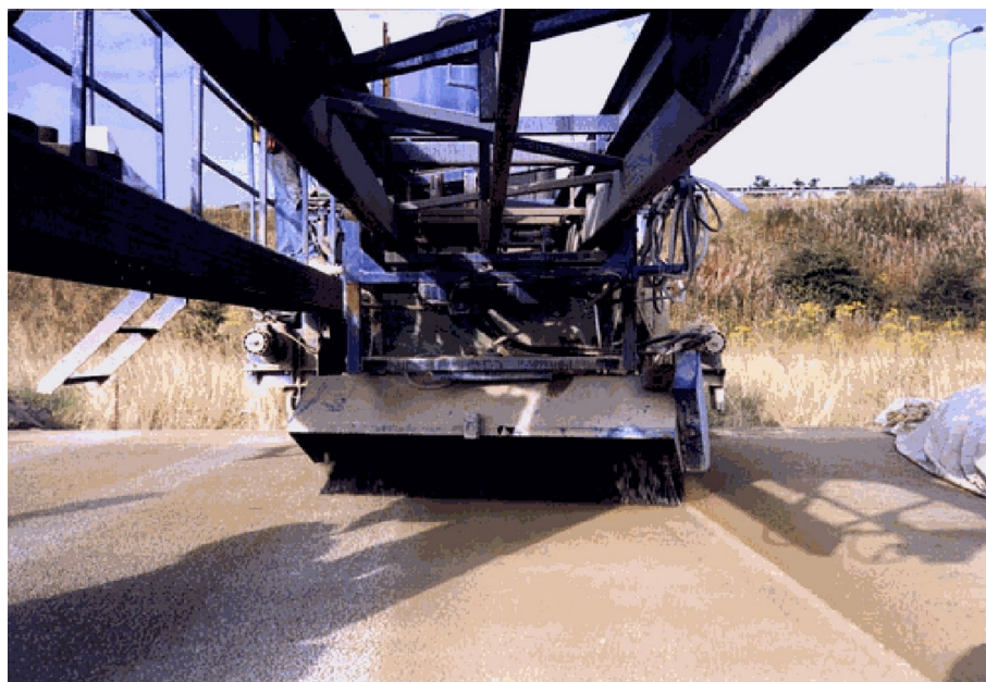
Figure 1: Brushing the surface to expose the aggregate.
