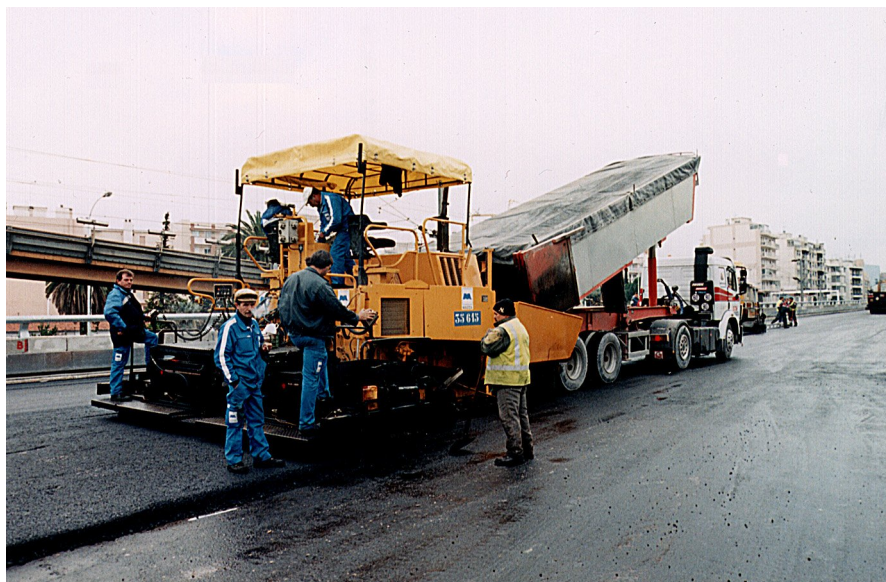
Figure 2: Laying of a noise-absorbing surface (noise reduction 3 dB(A)).
