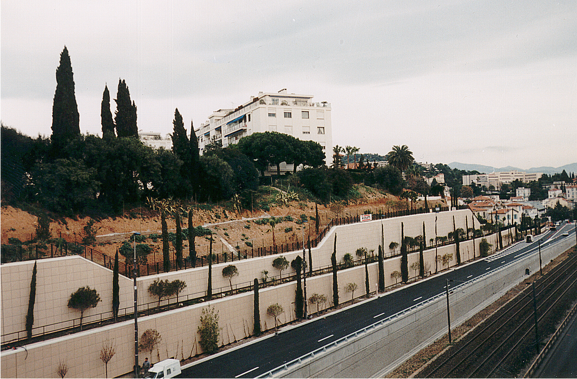
Figure 3: Noise reducing wall length 800 m cost: 4.5 MF (680 000 Euros).
