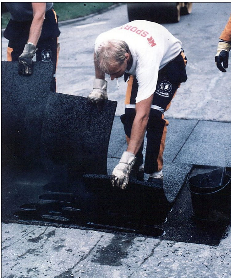
Figure 2: Panels of poroelastic material being laid on a street in Stockholm, in order to test durability over a winter season.
