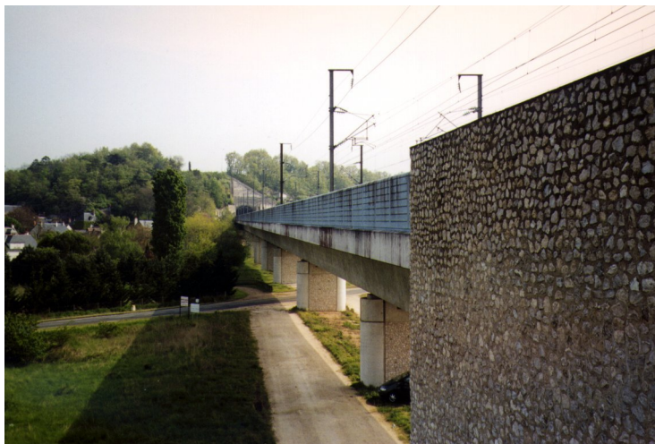
Figure 2: Viaduct at which noise measurements were recorded.
