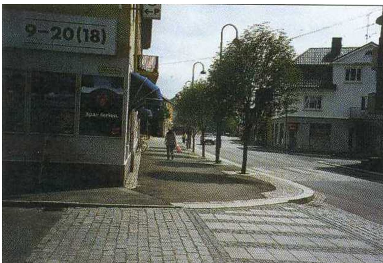
Figure 2: Pedestrian crossing with pavement stones.
