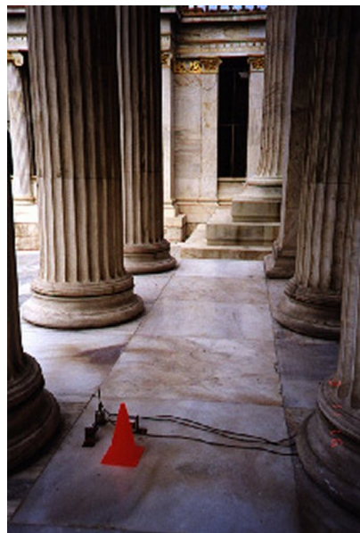
Figure 4: Point 5/Akademia building entry.
