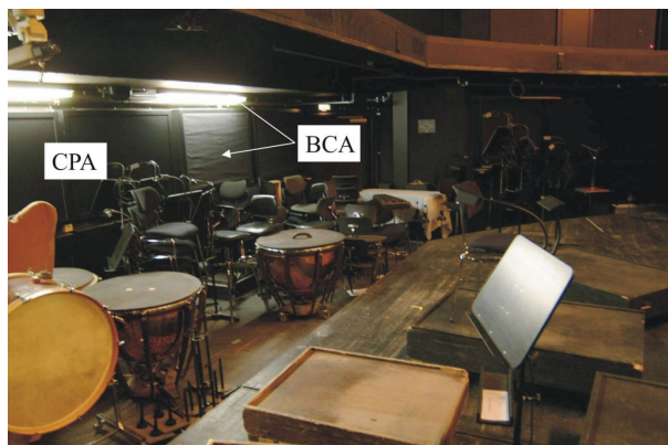
Figure 2: CPA and BCA mounted below the overhang in the pit of the Staatstheater Mainz.
