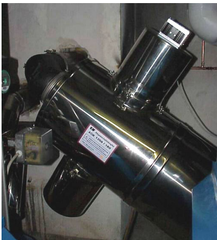
Figure 5: Aktiv+ Silencer [5] with additional reactive ( \lambda/4 ) branch resonator (photo: Kutzner+Weber).
