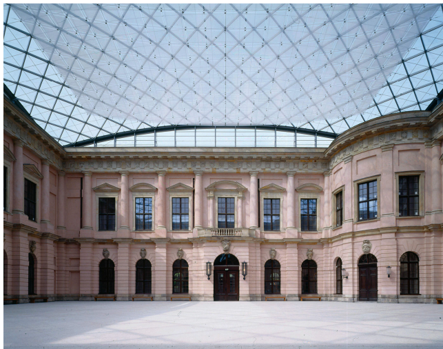
Figure 3: Transparent sail of micro-perforated foil under the new, concave-curved glass roof structure in the “Schlüterhof” of the DHM.
