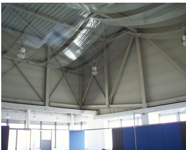
Figure 1: Freely suspended layers of micro-perforated foils in the "Forum" of the OIC.
