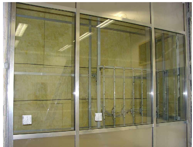
Figure 1: Reference façade at the test facility of Schueco in Bielefeld with the microphone array in the rear (right lower side).
