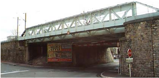
Figure 1: steel bridge GAVIGNOT selected for the study
