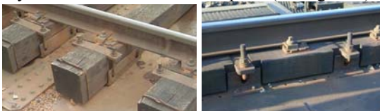
Figure 2: rail supported by sleepers or longitudinal sleepers
