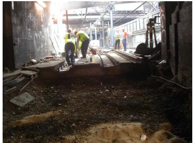
Figure 2: Entrance to the tunnel under the building; note the concrete structure in the background.
