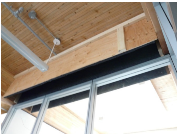
Figure 24 – The optimal U-shaped test silencer installed between the CIRS office and lab.
