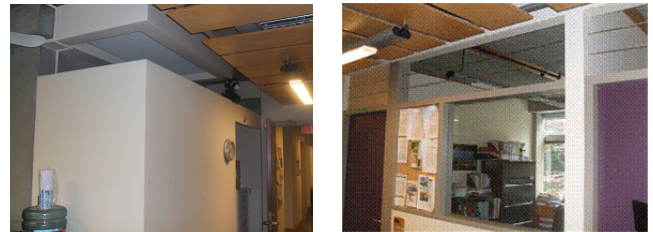
Figure 5 – Liu building natural-ventilation system: (left) shaft and floor openings; (right) office/corridor openings.
