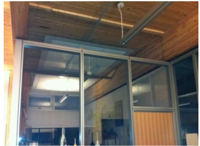
Figure 21 – Natural-ventilation opening in the partition between the office and lab in the CIRS building.
