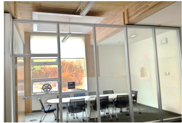
Figure 25 – Natural-ventilation opening in the partition between the lunch room and open-office area in the CIRS building.
