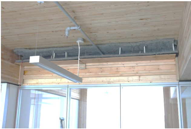
Figure 27 – The optimal Straight test silencer installed between the CIRS lunch room and open-office area.
