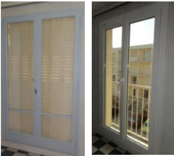
Figure 2. Example of mitigation solution, on the left single-glazed window without trickle vent, on the right double-glazed window with an acoustic trickle vent.
