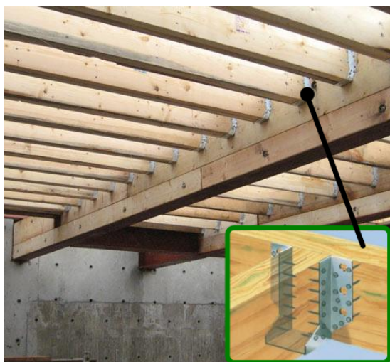
Figure 1: Wooden joist floor with wood connectors
