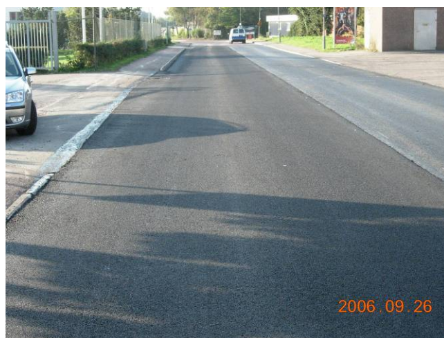
Fig. 2 Poroelastic asphalt pavement at Tagenevägen in Gothenburg.
