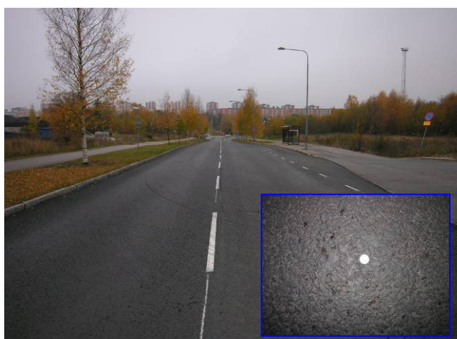
Fig. 5 Reference road surface type SMA 16 at Vandagatan in Stockholm. A Swedish 5 krona coin has been used in the close-up for reference.
