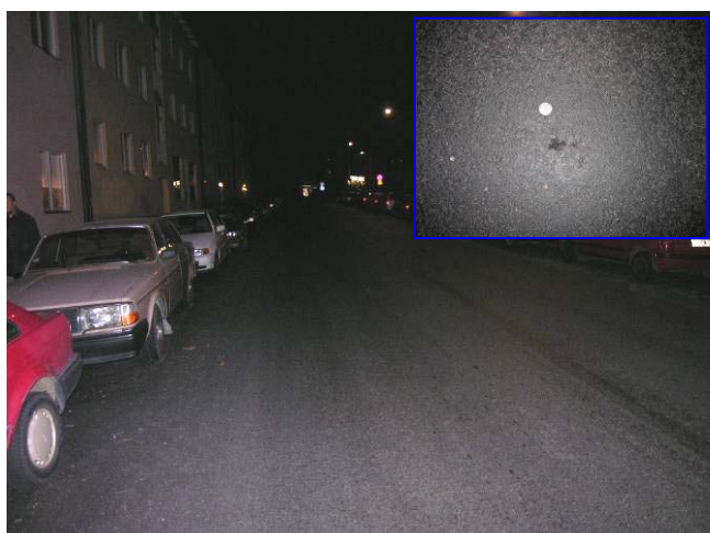
Fig. 6 Reference road surface type AC 16 at Tranebergsvägen in Stockholm. A Swedish 5 krona coin has been used in the close-up for reference.
