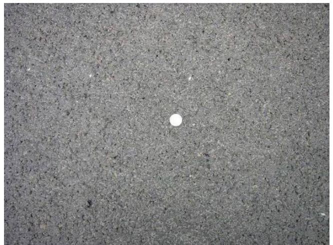
Fig. 3 Close up photo of the Thin Layer VIACOGRIP 8 with a Swedish 5 krona coin as reference.
