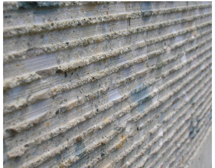
Figure 7: Example ground surface; conventional grind texture
