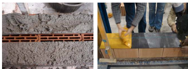
(a) Discontinuous joint (b) Adhesive band
