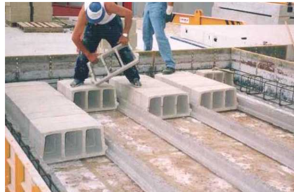
Fig. 1. Beam and block floor mounted in laboratory.
