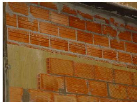
Fig. 3. Double ceramic brick wall.
