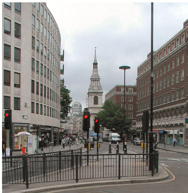
Fig. 3. The church steeple in Hune 2006. [Photo by authors]
