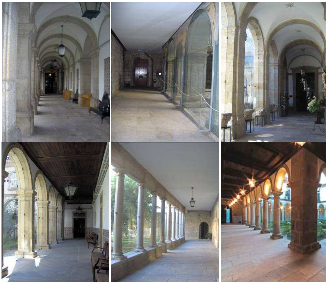
Fig. 1 to 6 The six studied cloisters with the rehabilitated galleries: openings between galleries and central yard closed with glass (top left to bottom right: BP, PSP, SB, ESE, SF, and CA) [3].
