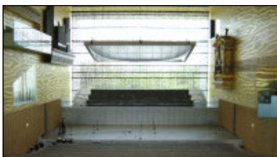
Fig. 4 CdM: canopy @ rear 8.6 m – front 10.0 m
