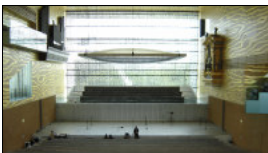
Fig. 2 CdM: canopy @ rear 8.6 m – front 8.6 m
