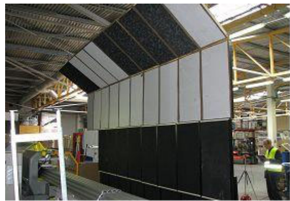
Fig. 6 General view of the acoustic partition wall in the workshop of aluminium pipe cutting
