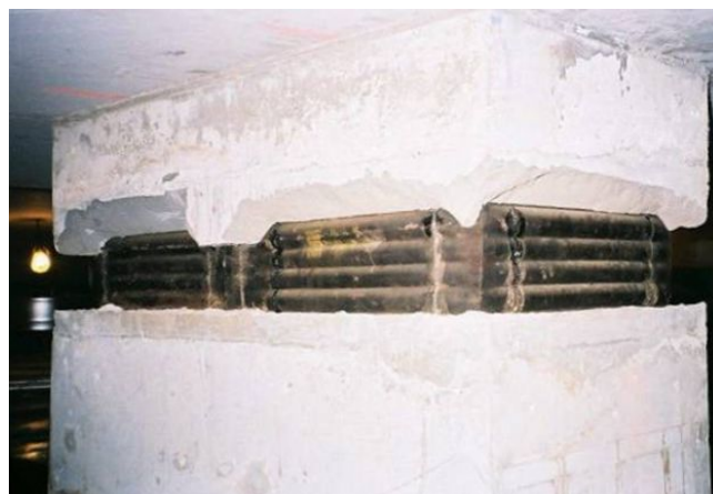
Fig. 6 Isolation Bearing Pads after Installation and Loading
