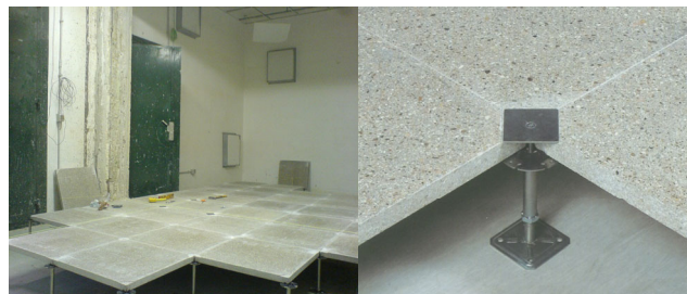
Fig.3: Sample mounting (left); particular of the panels and the support posts (right)
