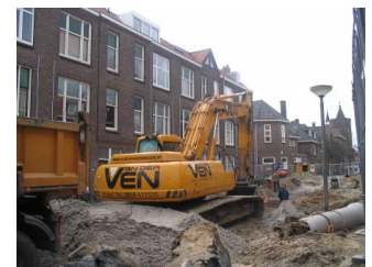
Figure 1b: Excavator working in a narrow residential street
