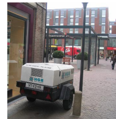
Figure 1d: Compressor in inner urban area
