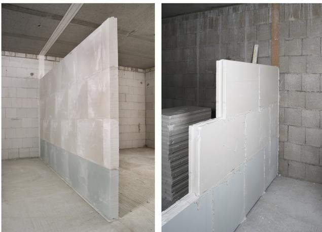
Fig. 1 - construction of gypsum walls in buildings
