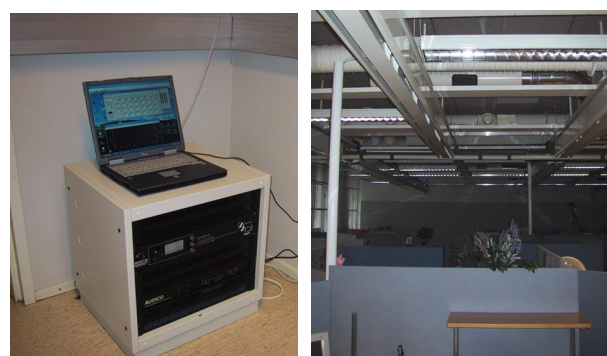
Fig. 1. Left) Central unit consisting of rack mounted signal generator and amplifier. The filters of the signal generator are configured with PC before launching. Right) One of the black loudspeakers installed above electric ceiling shelf.
