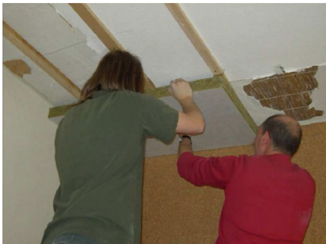
Figure 2: Replacing of parts of the ceiling in Schafisheim.
