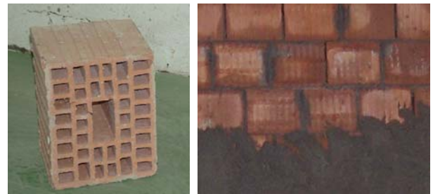
Fig.2 The brick of the flanking wall A (on the left) and the whole wall during the realization (on the right).
