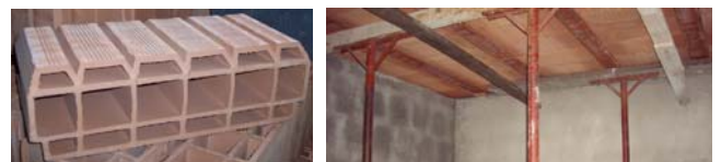
Fig.3 The blocks of the ceiling (on the left) and the whole tile-lintel floor during the realization (on the right).
