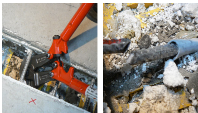
Fig. 8: Decreasing gradually the number of shear forces bars by intersecting the bars.
