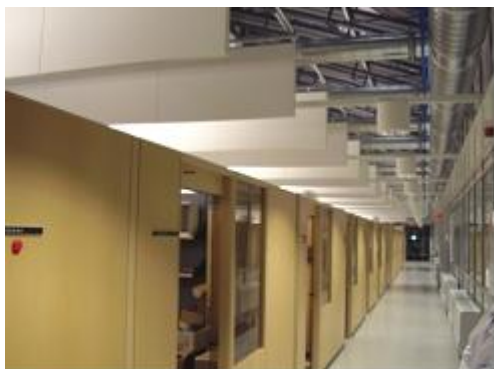
Fig. 1. Office 1 after the installation of hanging absorption baffles.
