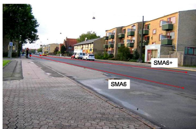
Figure 8: View of the measurement tracks at Kastrupvej -2
