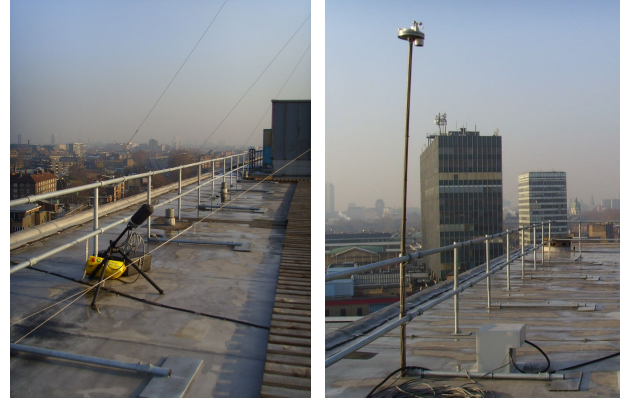
Fig 3. The roof-top monitoring equipment – noise, weather
