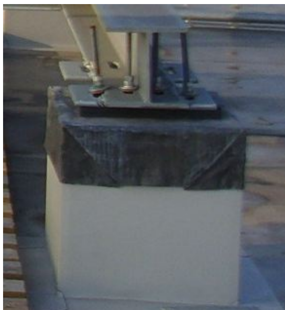
Fig 16. Turbine mounting uses vibration isolating pads
