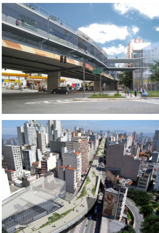
Fig. 2 and 3 Solutions for the “Minhocão”, proposed in 2003 by two architects, Juliana Corradini and José Alves, graduates from Faculty of Architecture and Urbanism of the University of São Paulo. Noise confinement is just one benefit. Annexed garage buildings, galleries, and a 60,000 m 2 traffic-free area on top, for pedestrians and leisure, are other inputs for urban revitalization downtown.
