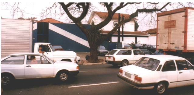
Fig. 4: Residences transformed into office buildings, in a highly noisy street. The cheapest solution was to move windows to the back and make a wall façade in front. The blue building gave the idea and the white one copied it.
